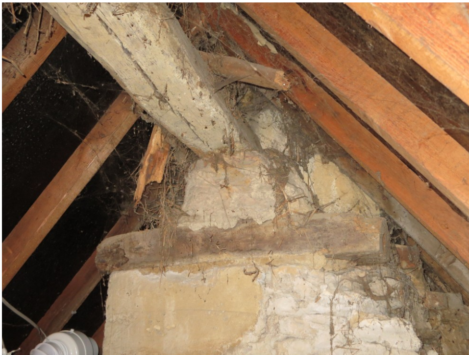
The surviving ridge beam at the west end, with timber plate to chimneystack
