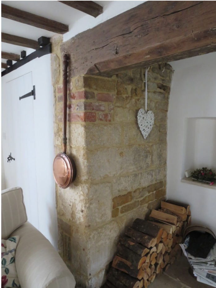
The inglenook fireplace, with raised beam and brick blocking
